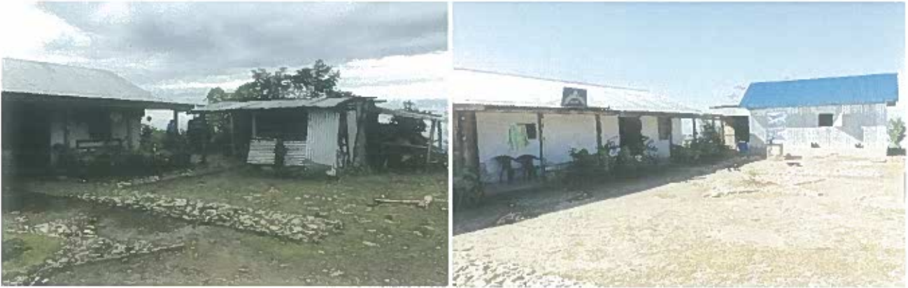
Jorpokhari (Panchthar) Police Post building before and after renovation
